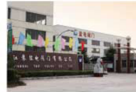
GGC Valve Plant
