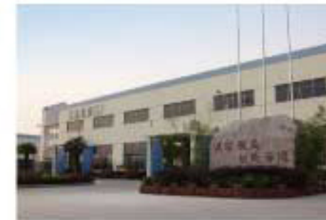
Ball Valve Plant
